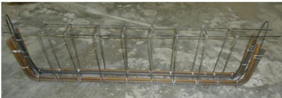
**Fig .(1) Steel reinforcement cage**
